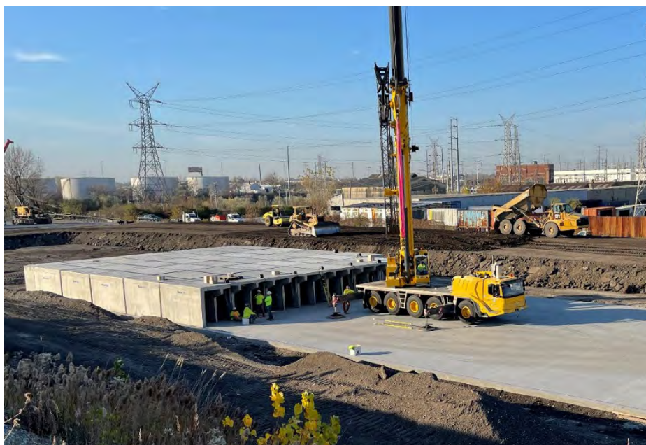
Underground stormwater trap #1
