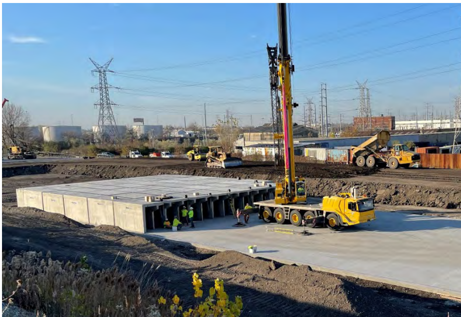
Underground stormwater trap #1
